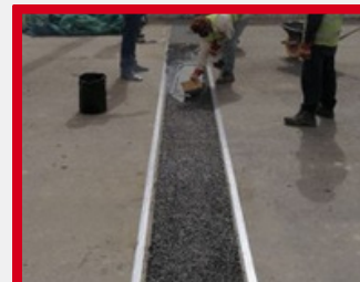
Sealing joint surface
