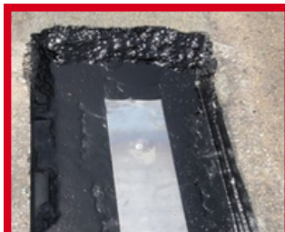
Installing steel plates
