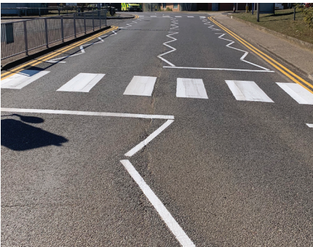
Lifeline® A highly reflective white thermoplastic that can be applied by screed, extrusion or spray. It offers multiple retroreflectivity and performance levels, with all grades certified on UK road trails.
