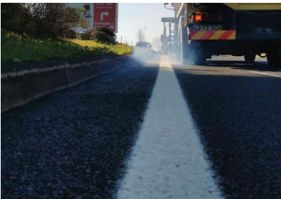
Thermaspray™ A spray-applied thermoplastic in white and yellow, with reflective and non-reflective options. Suitable for warmer climates, it is designed for high-volume marking. Certified for highways and applied using specialist spray technology.
