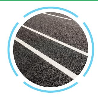
Also suitable for post-spraying with glass beads and/or antiskid material to enhance night visibility and skid resistance.
