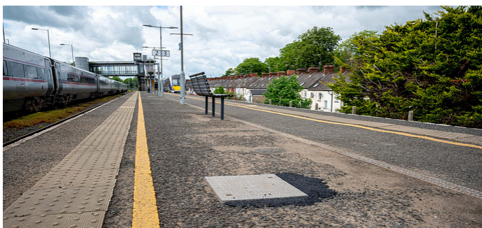
The aged platform surface was pitted and spalled.
