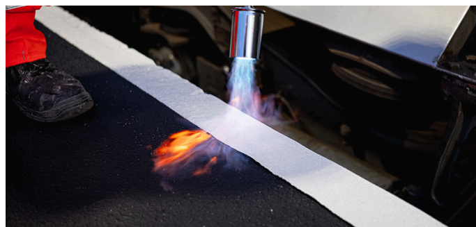
Prismo® Regulatory Preformed Thermoplastic was used to delineate the platform edge.
