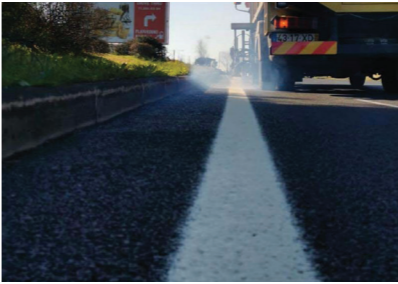
Sprayplastic® A spray-applied thermoplastic in white and yellow, with reflective and non-reflective options. Suitable for warmer climates, it is designed for high-volume marking. Certified for highways and applied using specialist spray technology.
